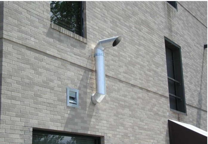
Typical side wall exterior vent exit
