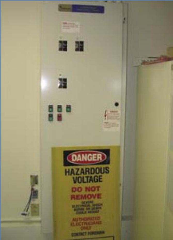
Figure 43 - Main Disconnect Panel or Power Distribution Box
