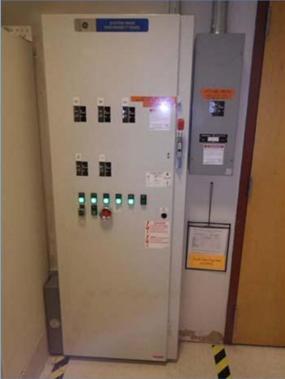
Figure 22 - Innova Main Disconnect Panel
